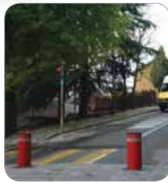
Entry driveway to public buildings
