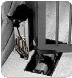
Installation with motor-pump and jack - internal view
