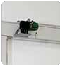
Installation of MEC 200 LB on a sliding door
