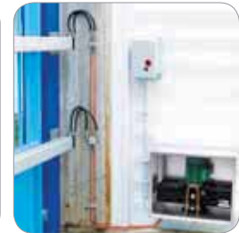
Oil-hydraulic motor-pump MEC 700/80 VENTIL double-tank inside the enclosure
